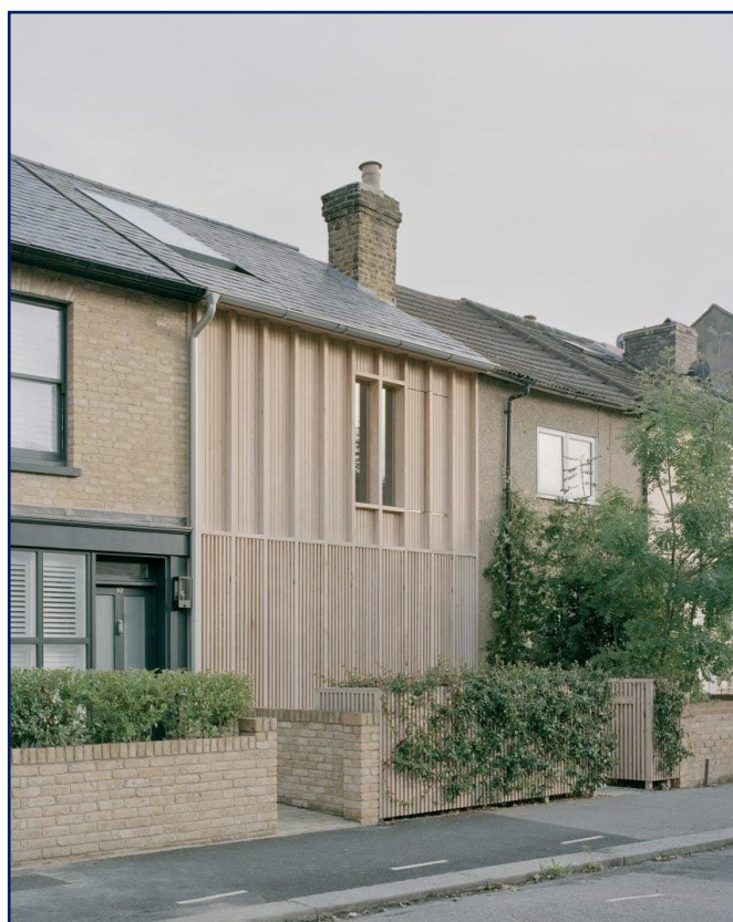
Spruce House by architects ao-ft is located in a conservation area in Walthamstow, London. The house is built with cross laminated timber. Image courtesy of ao-ft
